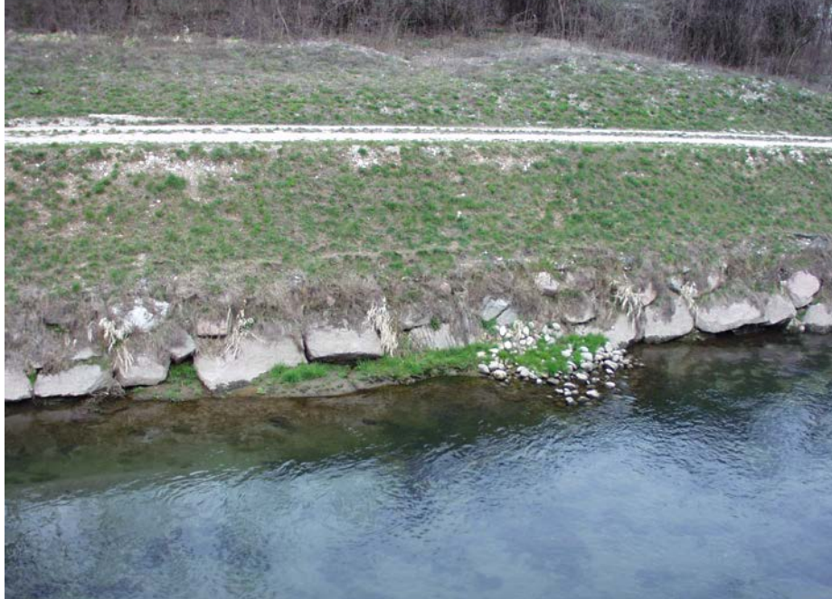
Fig. 13: Embankment stabilisation with the Krismer System® (03/2004)
