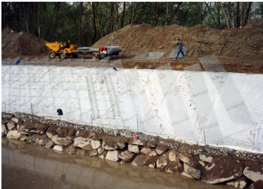
Fig. 9: Laying the segments of the J.K.S. panels crosswise to the fall line of the embankment and against the flow direction of the watercourse
