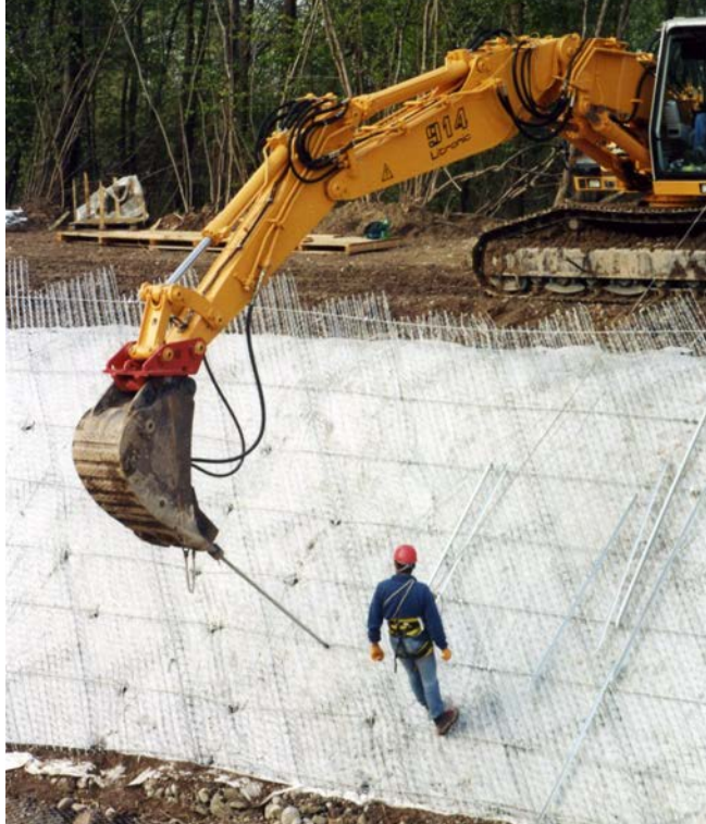
Fig. 10: Ramming the ground nails
