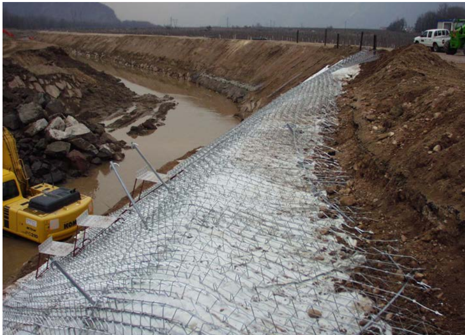
Fig. 11: Integration of the Krismer System® into the adjacent area (top border zone)
