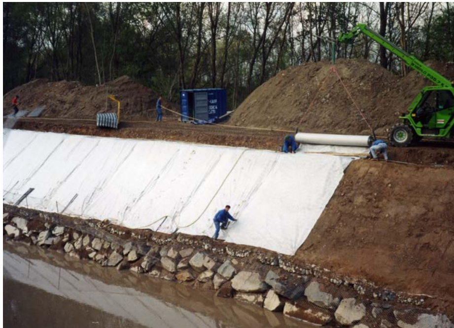
Fig. 7: Installation of the geotextile on the embankment surface
