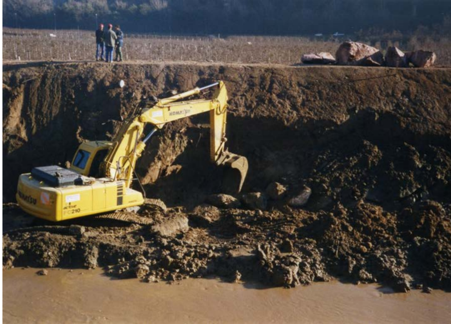
Fig. 4: Placing of the river stones (riprap)
