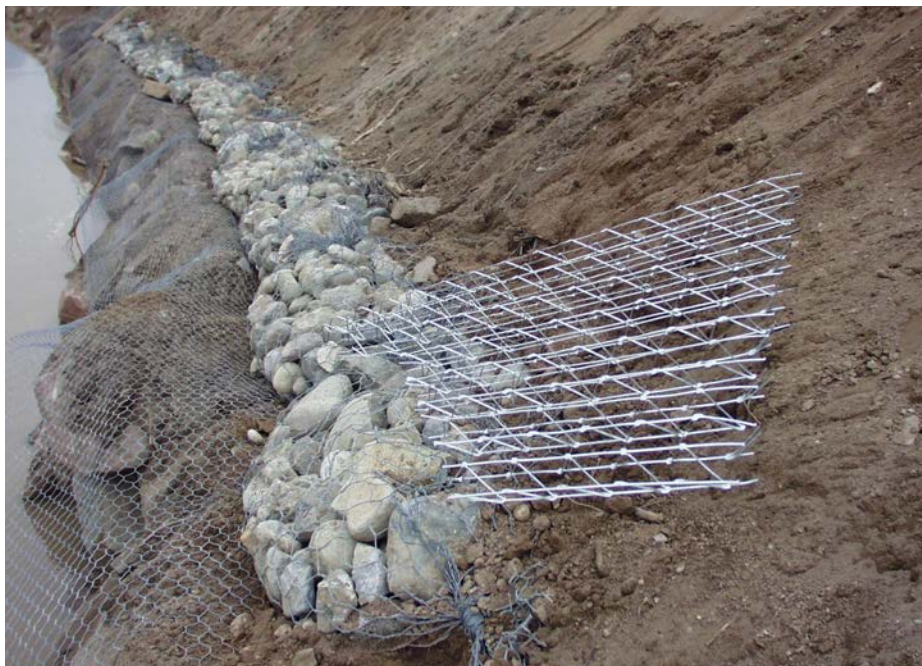
Fig. 5: Integration of the Krismer System® at the embankment base
