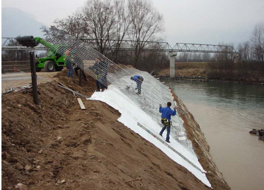
Fig. 8: Installation of the J.K.S. panels, pre-assembled into larger segments
