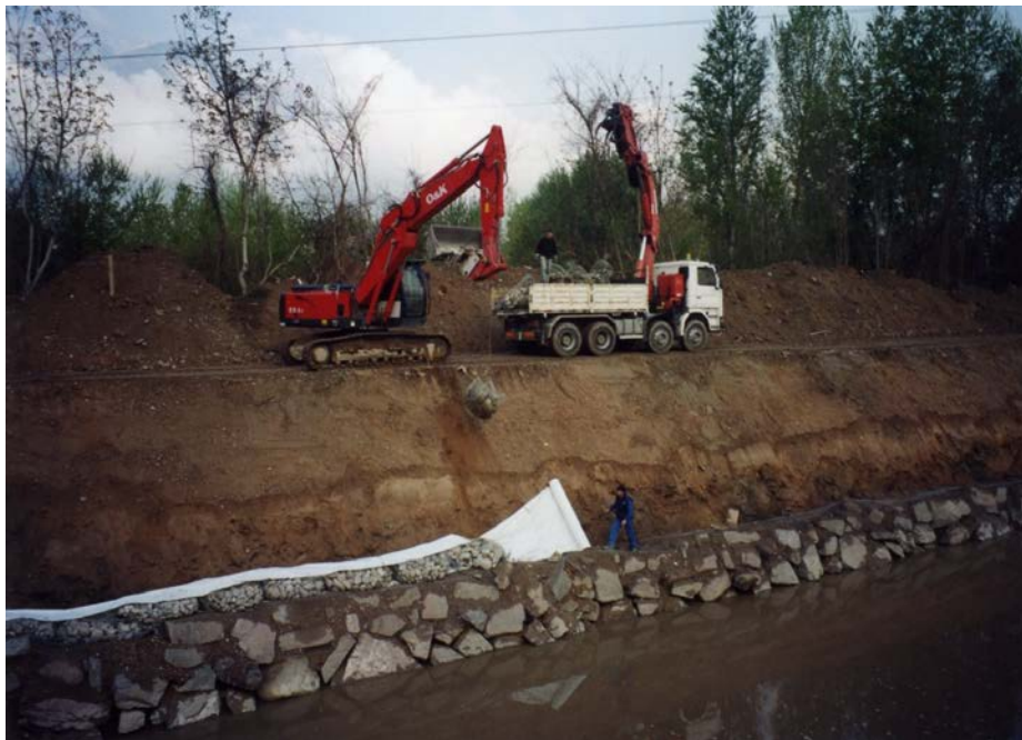
Fig. 6: Wire netting, geotextile and sack gabions were used for the integration of the Krismer System® at the embankment base
