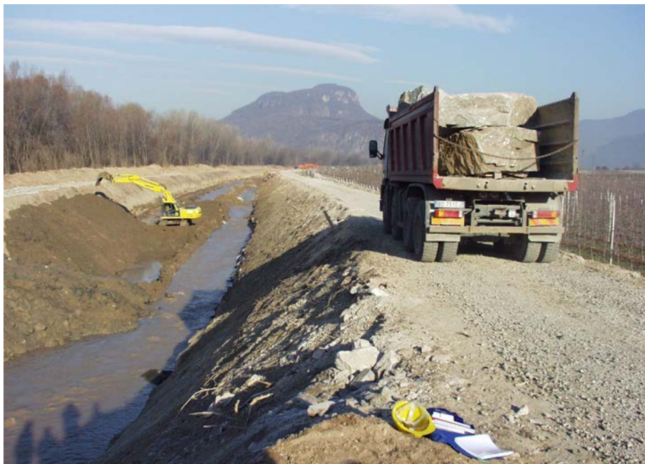
Fig. 3: Delivery of river stones for the construction of a riprap stone wall for the integration of the embankment in the base of the channel
