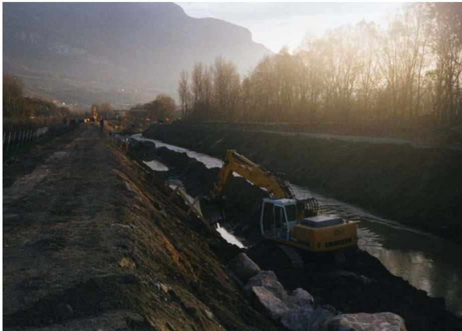
Fig. 2: Widening of the existing riverbed and constructing of the required embankment inclination
