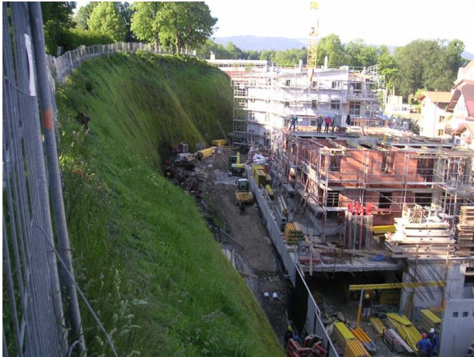
Abb. 15/16: Integration of the Krismer System® approx. 1.50 m over the top of slope into the surrounding terrain
