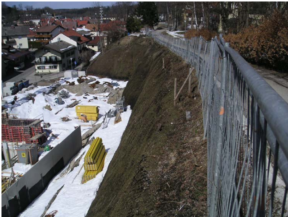
Fig. 11/12: Cut slope, Spring 2006 - The topsoil was applied onto the slope surface using the wet spraying method. Seeds were mixed into the humus during its application.
