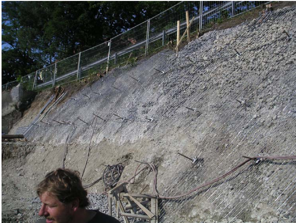
Fig. 5: Second excavation step, immediately followed by stabilisation of the slope
