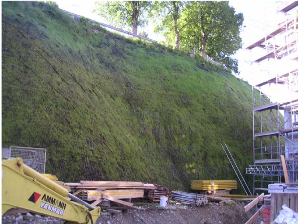
Fig. 13/14: State of the slope in June 2006, surface covered with germinating plants
