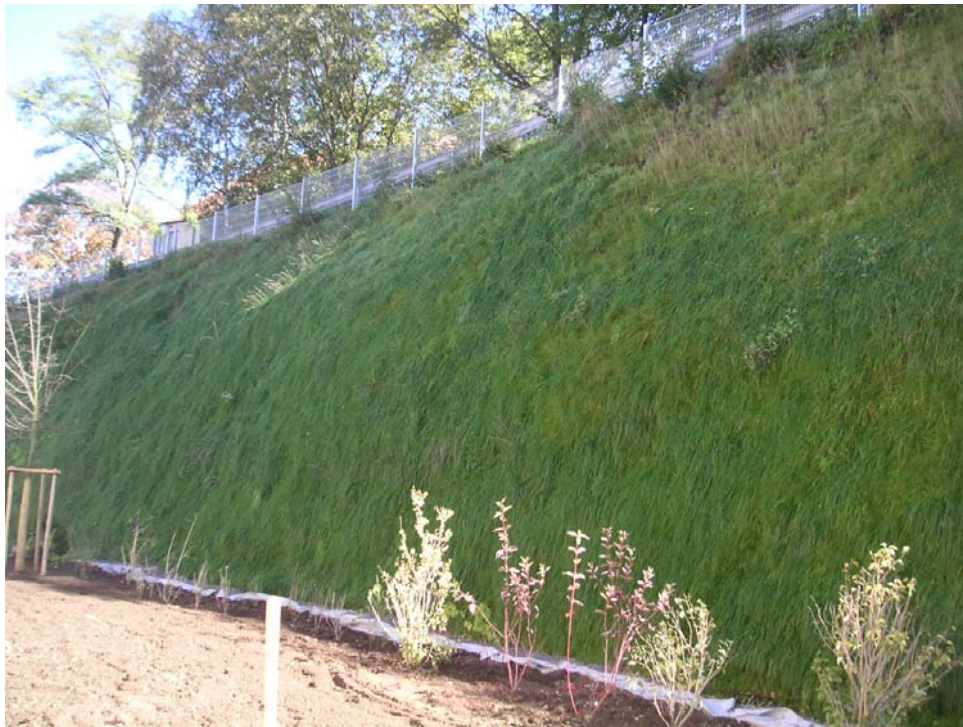
Fig. 20: Finished cut slope combined with to neighbouring gardens
