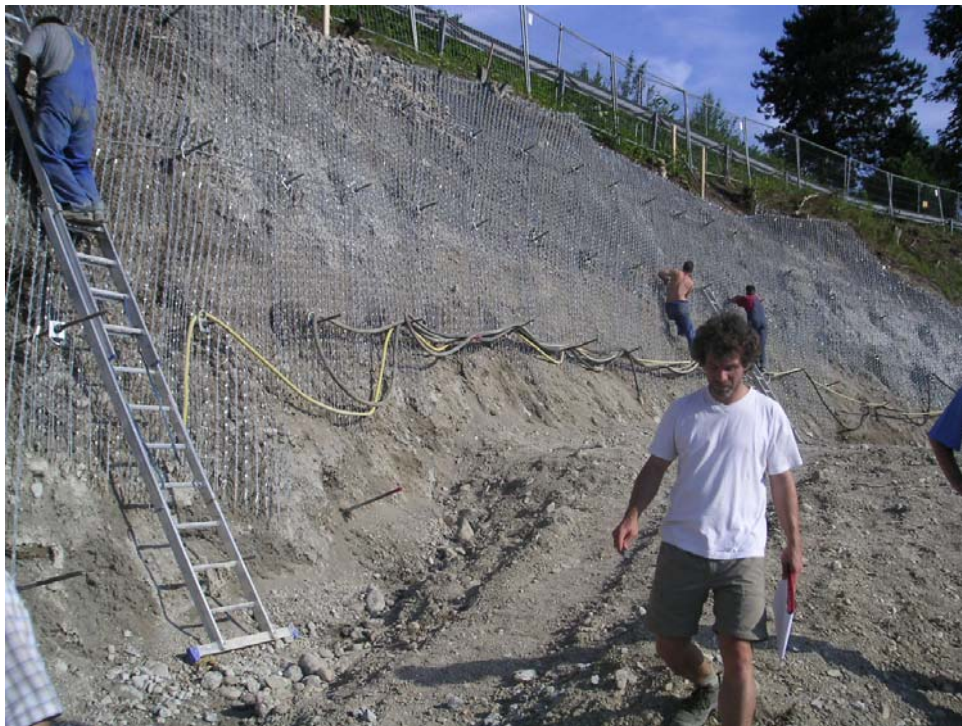
Fig. 4: The excavation work is immediately followed by the stabilisation work for the slope, done from the interim berm
