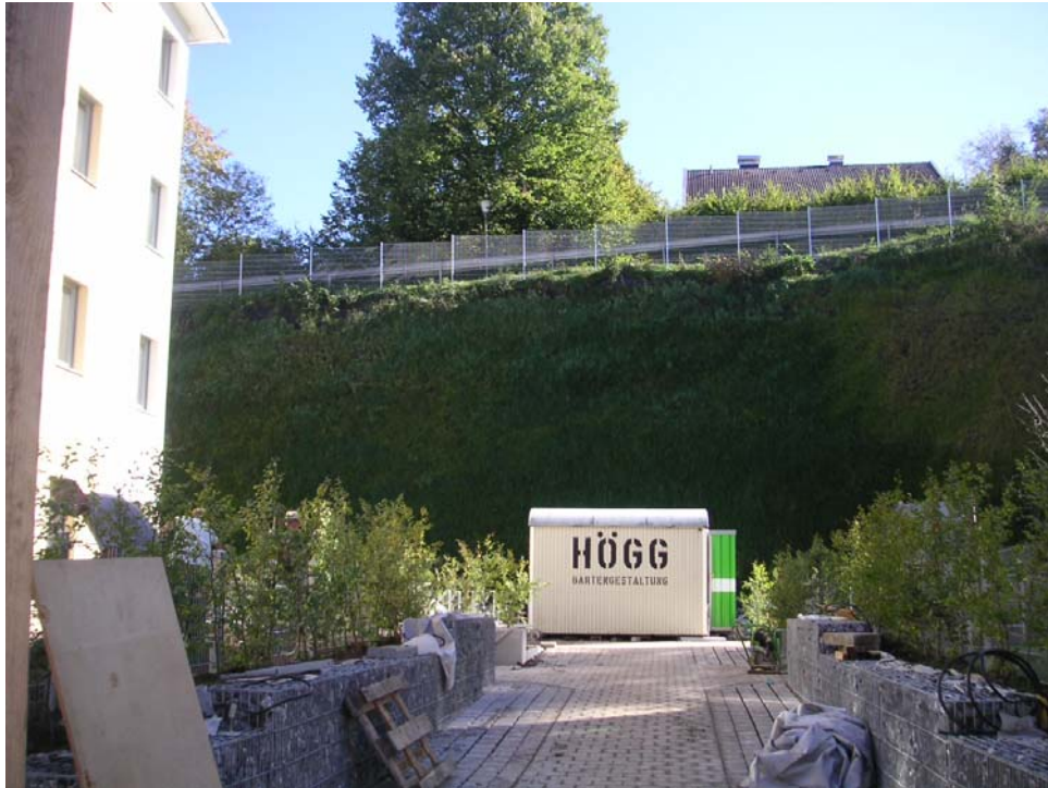
Fig. 19: State of the slope in October 2006
