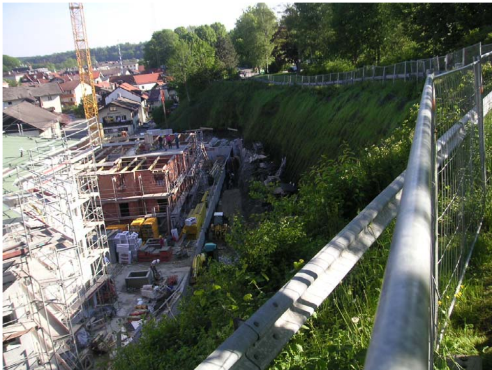
Abb. 15/16: Integration of the Krismer System® approx. 1.50 m over the top of slope into the surrounding terrain
