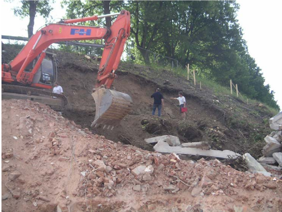
Fig. 3: First excavation step, excavating the new 65° cut slope in stages
