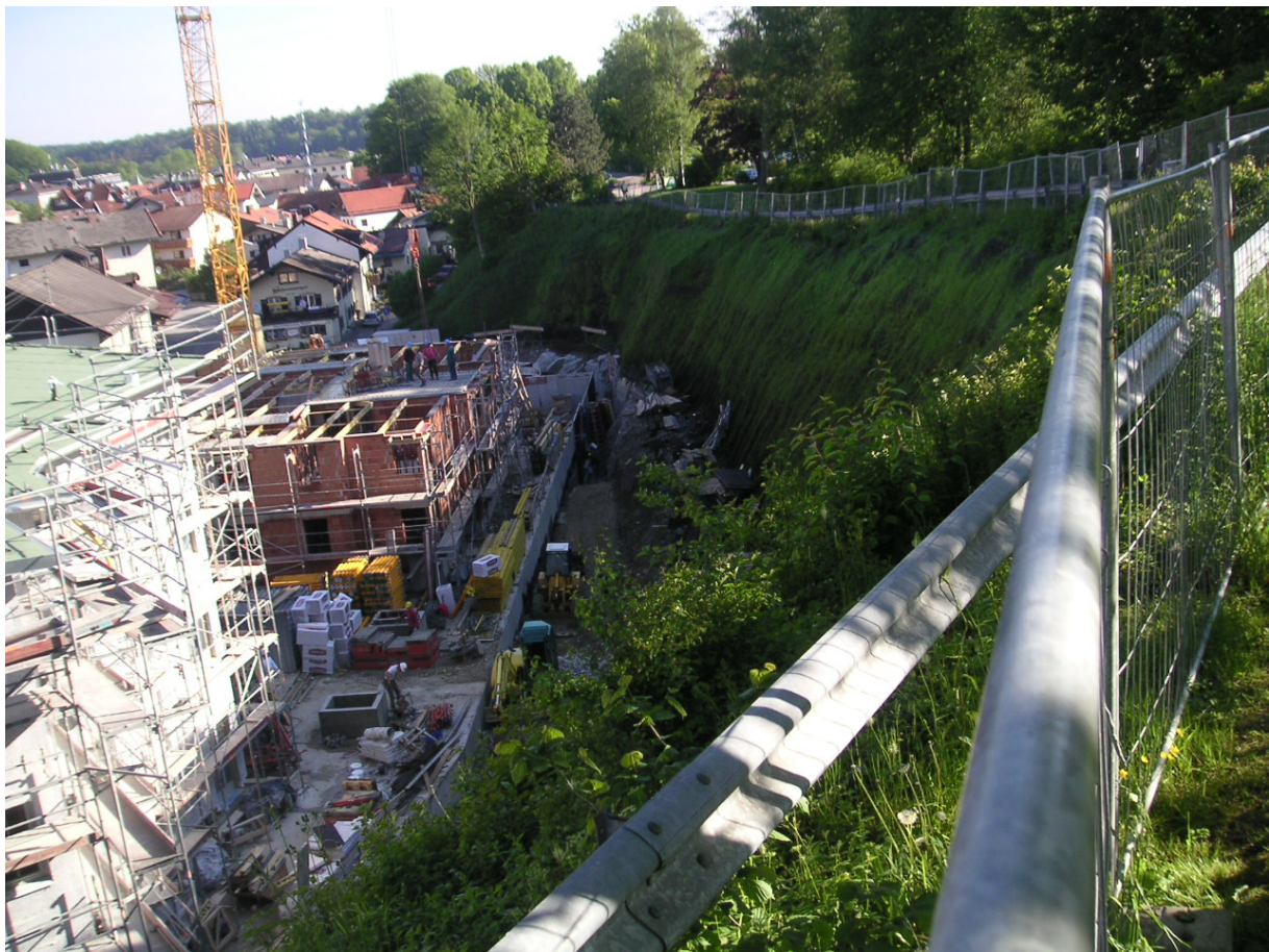
Fig. 1: Finished slope stabilisation
