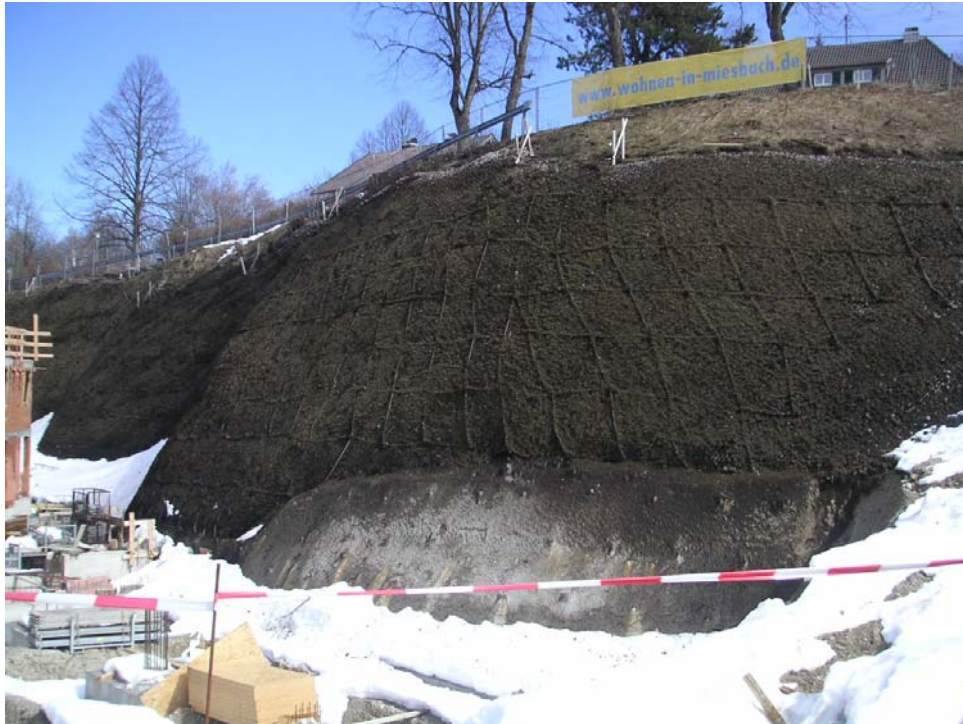
Fig. 11/12: Cut slope, Spring 2006 - The topsoil was applied onto the slope surface using the wet spraying method. Seeds were mixed into the humus during its application.
