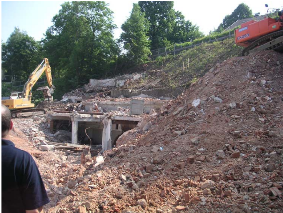
Fig. 2: Initial situation - demolition of the old dairy
