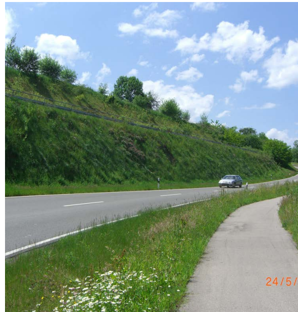
Fig. 7-8: Slope stabilised with the Krismer System®: 1 year (Fig. 7 - left) as well as 6 years (Fig. 8 - right) after the installation was completed
