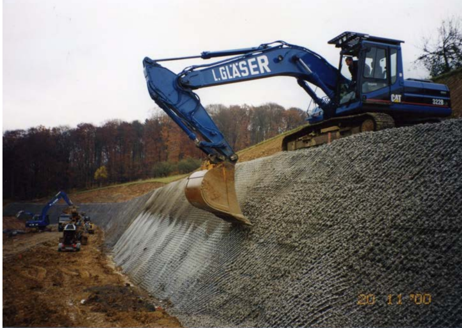
Fig. 4: Gravel filling (grain size: 32/60 mm)
