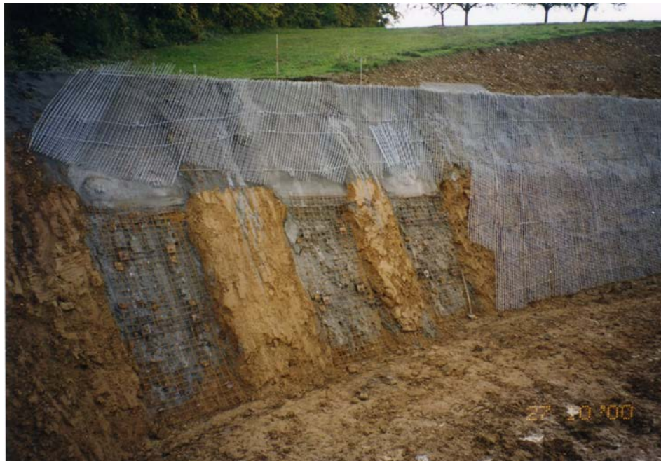
Fig. 3: Areas which were pre-stabilised with shotcrete and GEWI anchors
