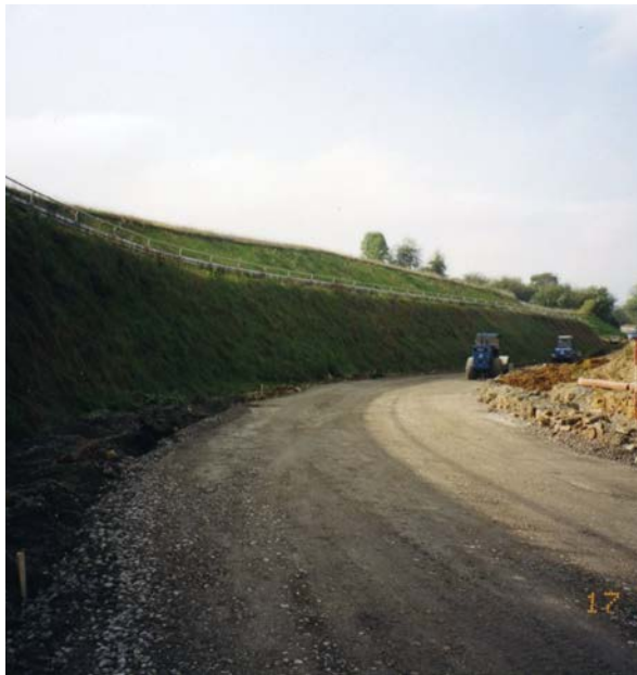
Fig. 7-8: Slope stabilised with the Krismer System®: 1 year (Fig. 7 - left) as well as 6 years (Fig. 8 - right) after the installation was completed
