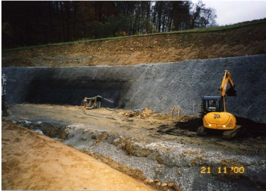
Fig. 6: Filling the top soil by means of a spraying machine
