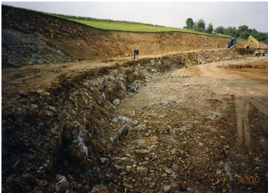
Fig. 1: Earth movement work for the new K 1897 county road
