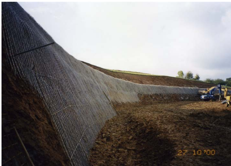
Fig. 2: Installation of the Krismer System® in several steps
