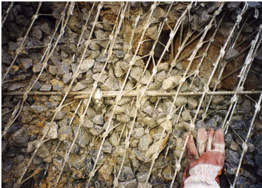
Fig. 5: J.K.S. panel with gravel fill
